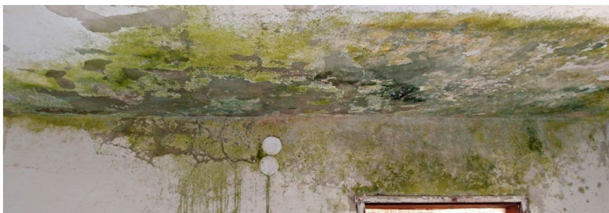
FIGURE 27 Commonly seen mould and humidity (Photo from Sisak-Moslavina County in Croatia)
